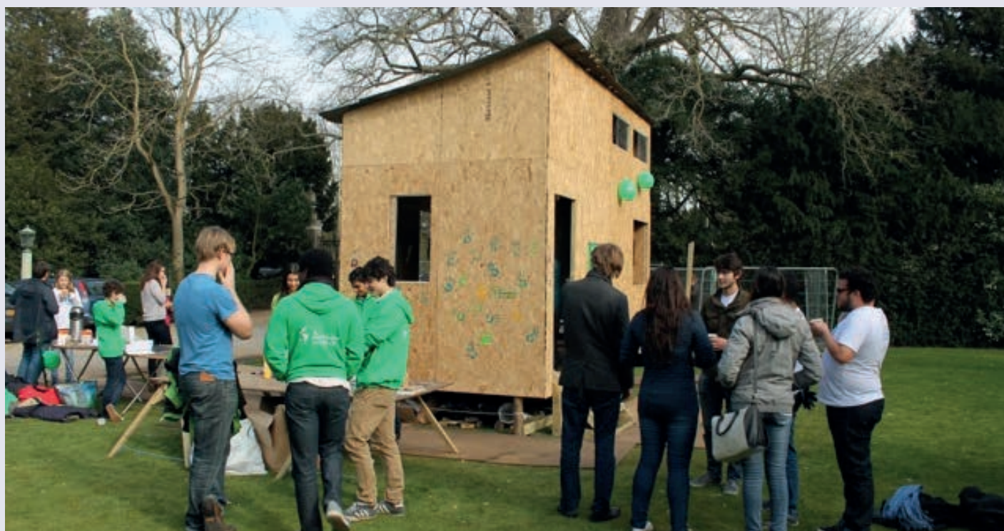
Eco-House prototype taking shape on the front lawn of Memorial Court
