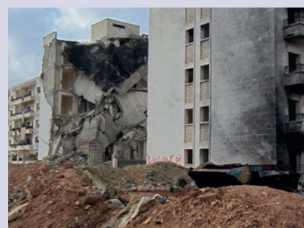
Bomb damage in Aleppo
