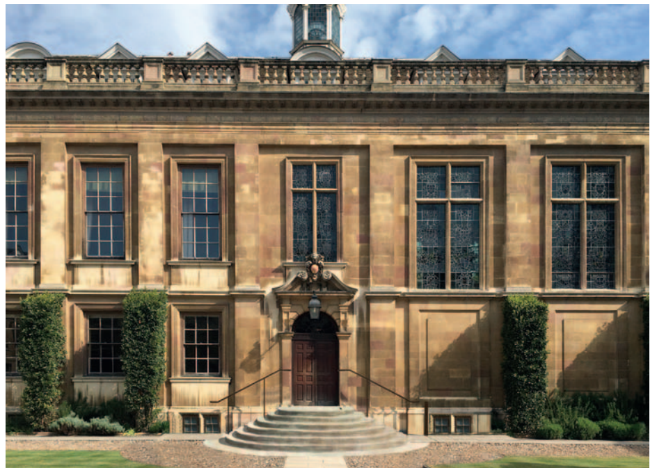
Proposed view of the entrance to H staircase. Almost unchanged, with concealed platform lift in steps
